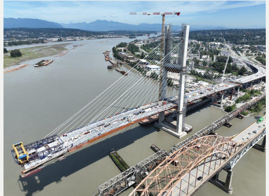
Photo 2: Concrete overlay main span to South Approach
