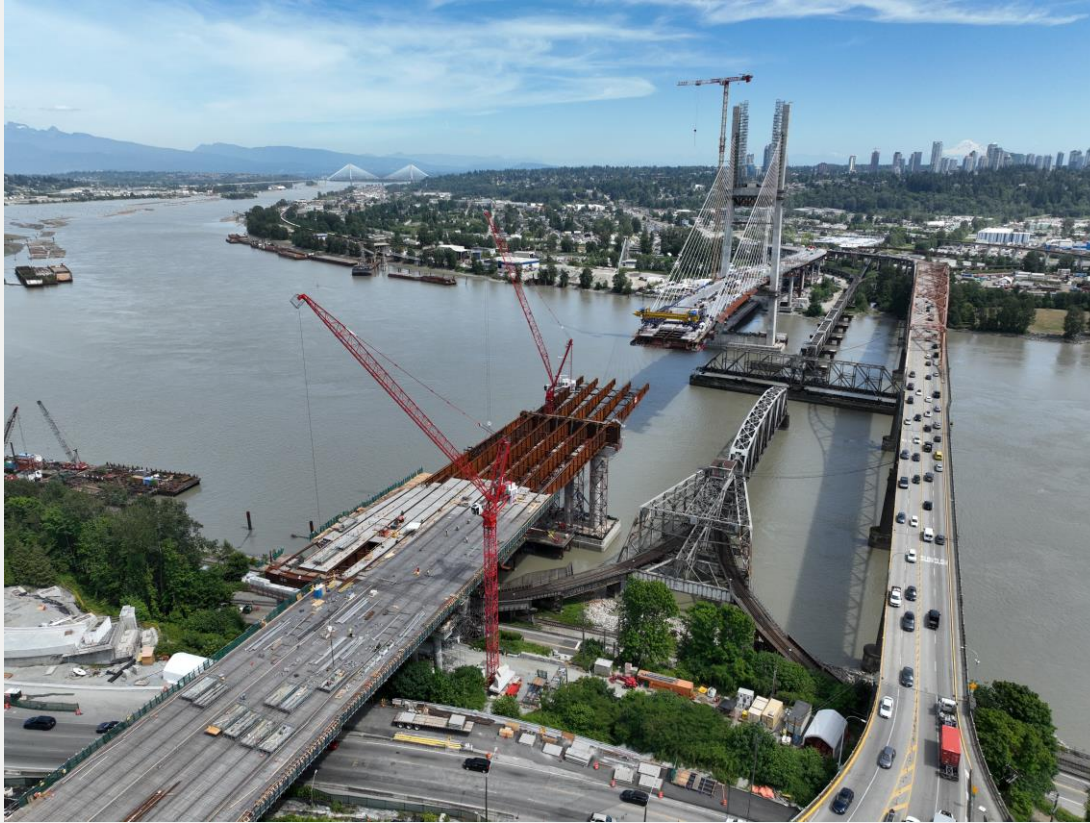
Photo 5: Ongoing girder and panel installation for the North Approach
