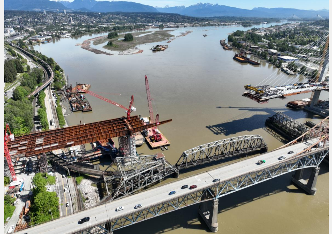
Photo 6: Ongoing girder and panel installation for the North Approach
