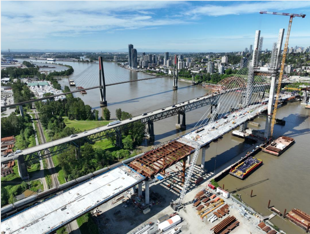
Photo 3: South Approach-end span- main span connection and cable stay installation ongoing
