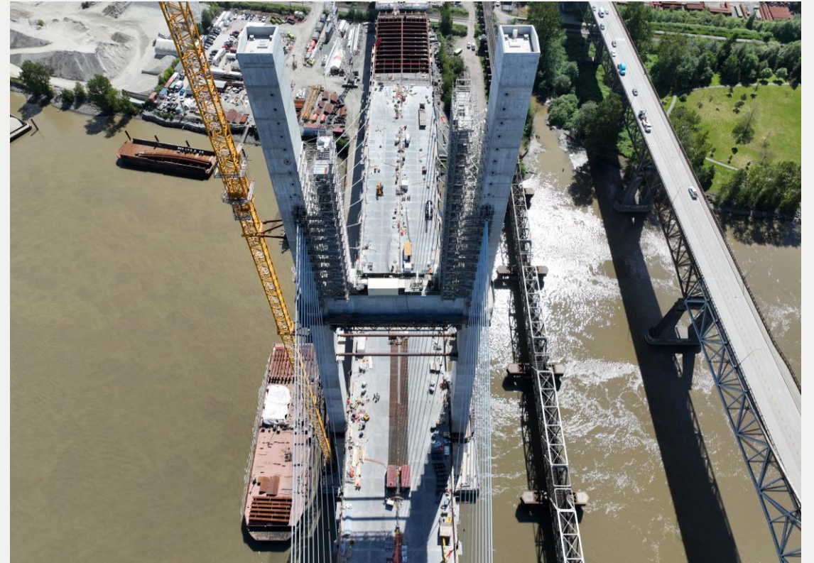
Photo 4: South Approach-end span deck panel installation and concrete overlay
