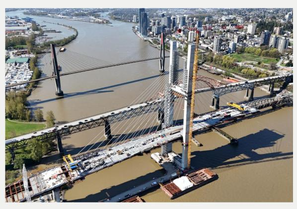
Photo 2: Concrete overlay main span to South and North Approach
