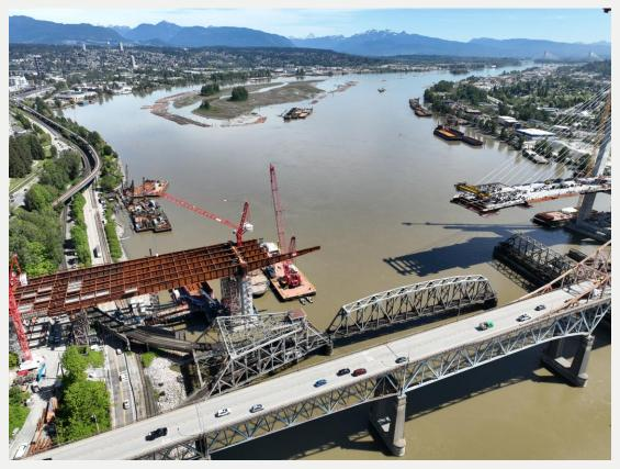
Photo 5: North Approach connection to main span (SM-011) ongoing
