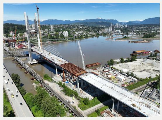
Photo 3: South Approach-end span- main span connection and cable stay installation
