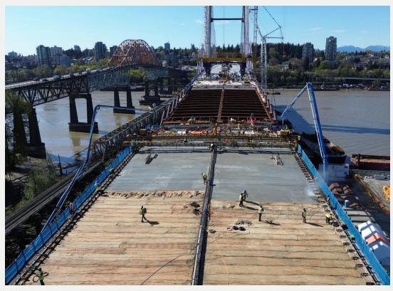
Photo 4: South Approach-end span deck panel installation and concrete overlay
