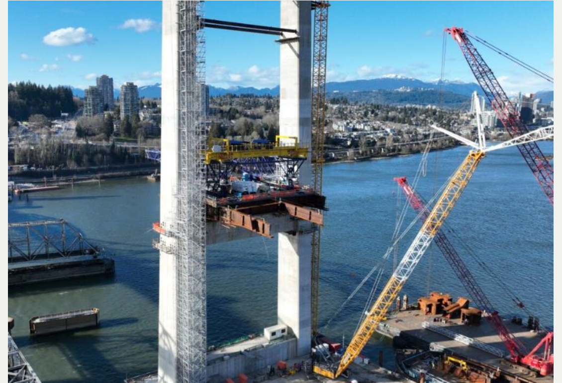
Photo 6: Pier S1 gantry and ongoing bridge deck construction
