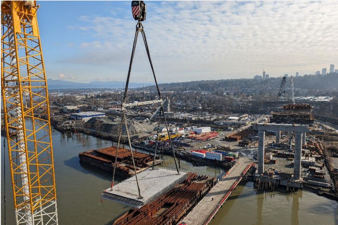
Photo 5: Lifting of bridge deck panel
