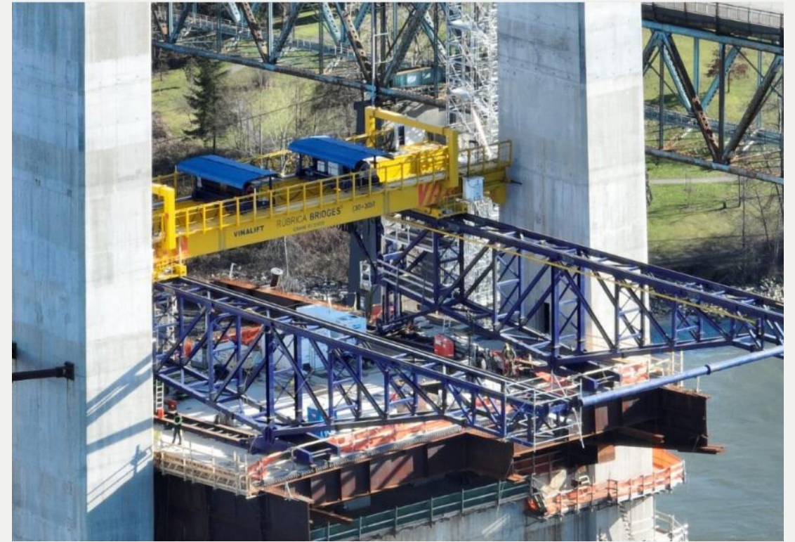
Photo 4: Pier S1 gantry close-up
