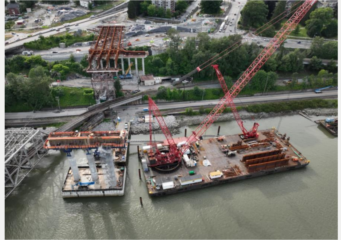
Photo 6: N1 Pier Cap construction, looking north
