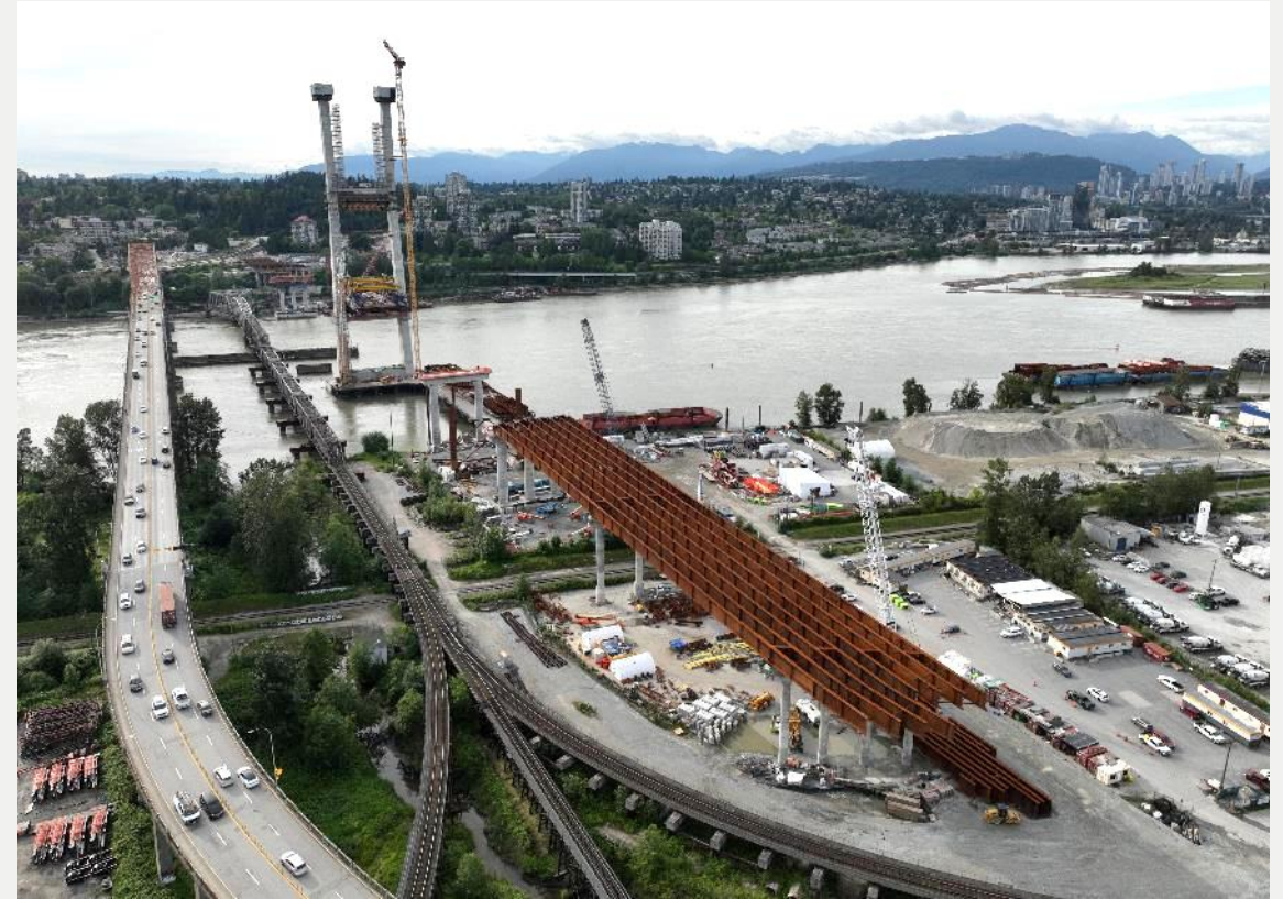
Photo 4: Looking northeast towards Pier S1
