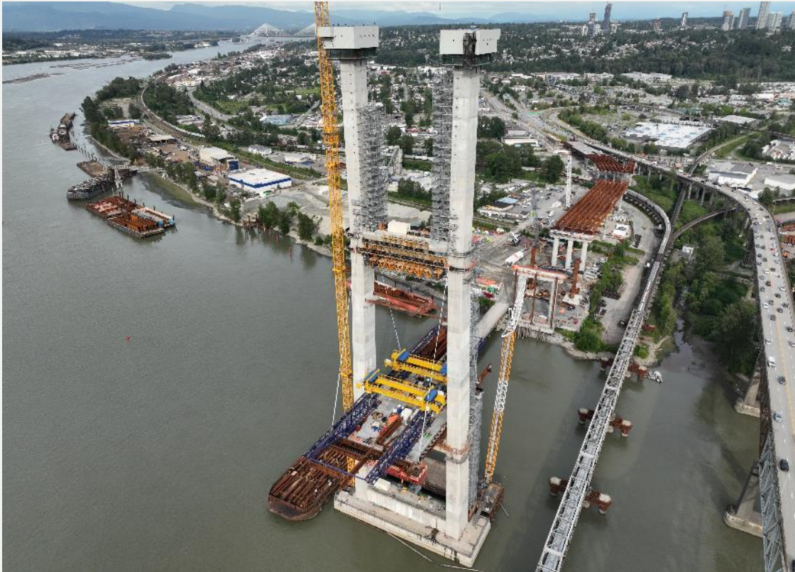
Photo 1: Pier S1, looking northwest
