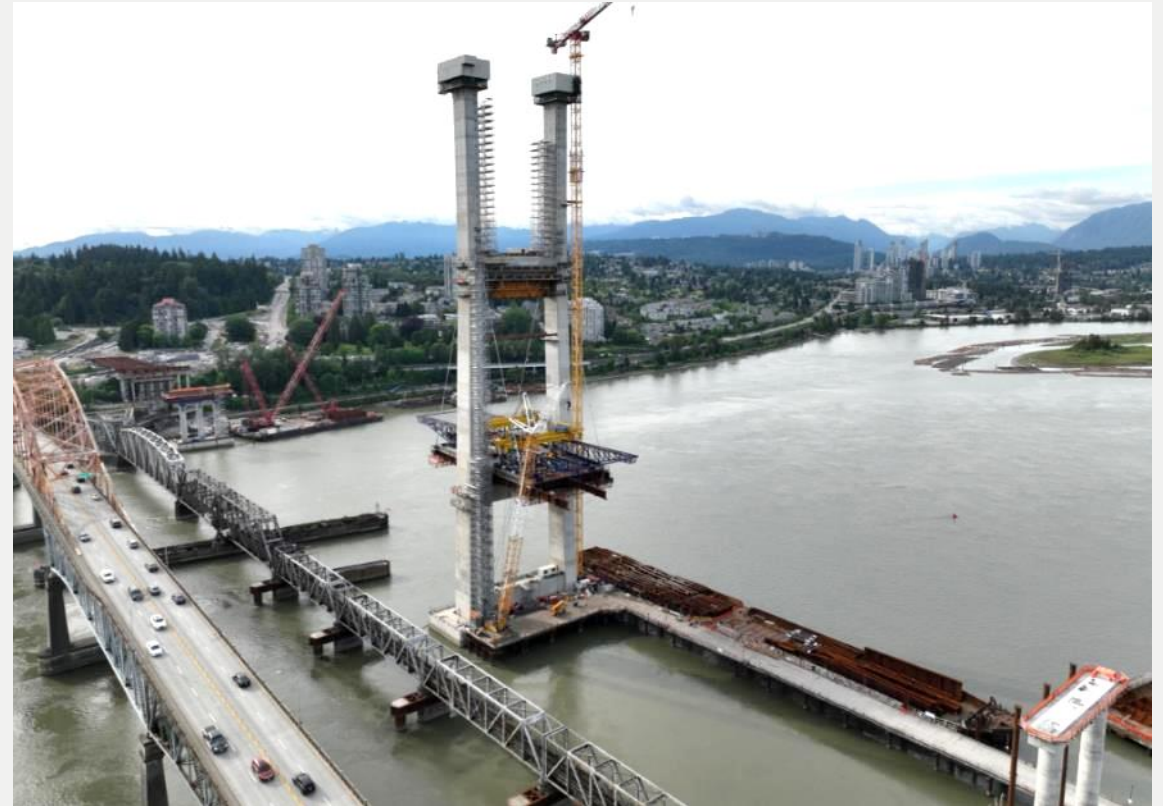
Photo 2: Pier S1, looking northeast
