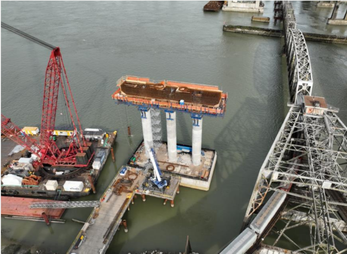
Photo 5: N1 Pier Cap construction, looking south
