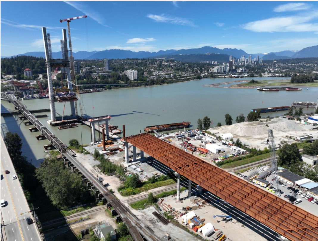
Photo 3: Pier S1, looking north – South Approach girder installation progressing
