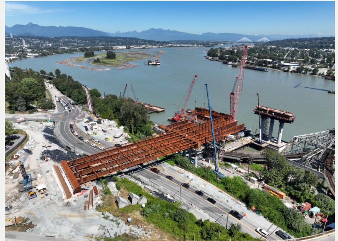
Photo 6: Ongoing girder installation for the North Approach
