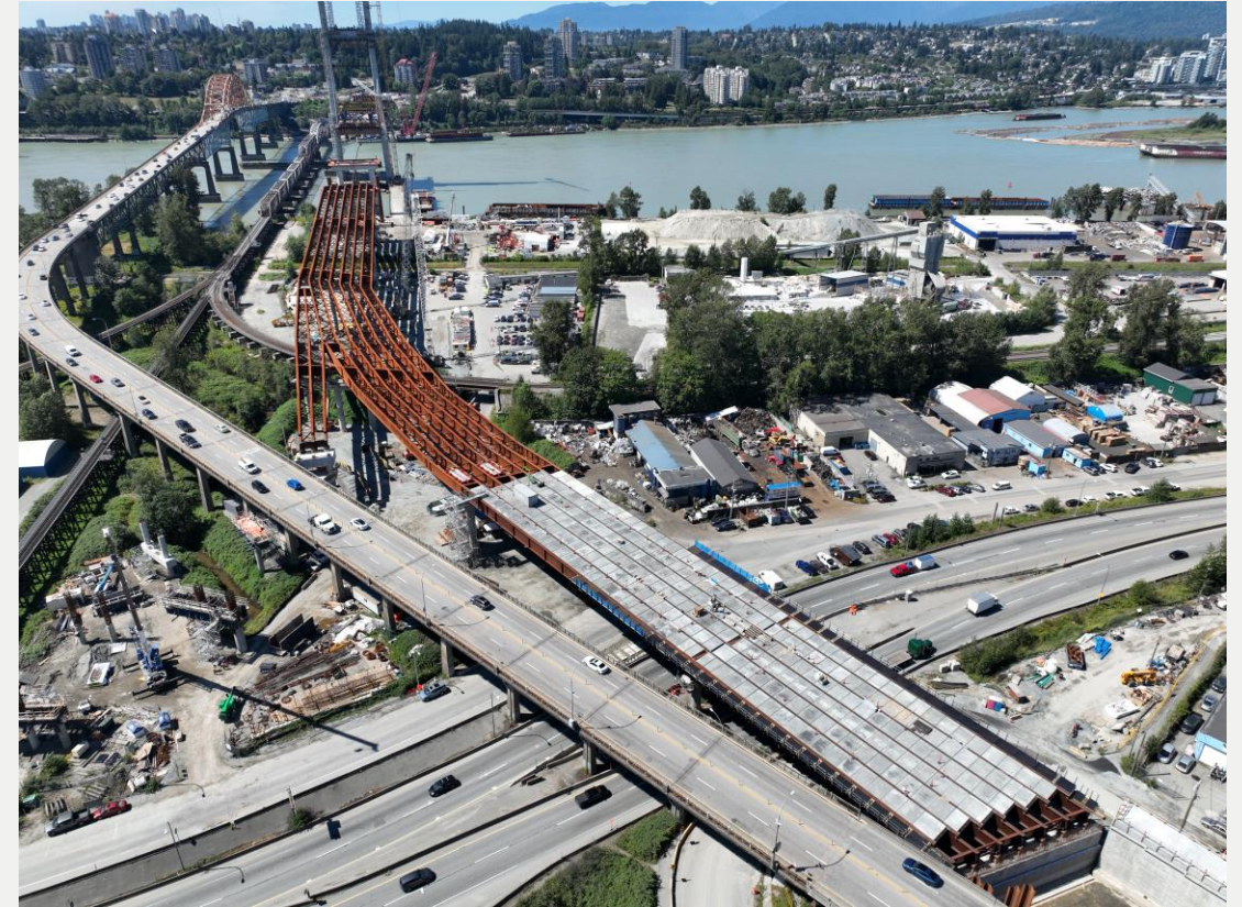
Photo 4: South Approach - Deck panel installation across Highway 17
