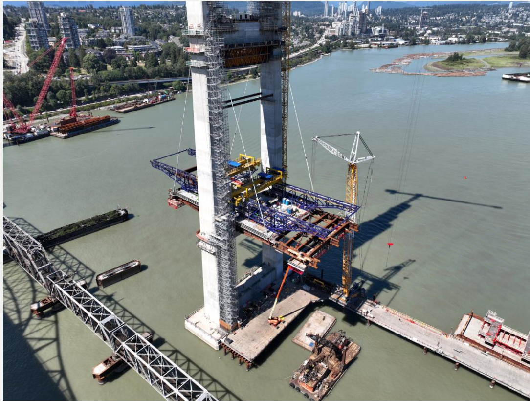
Photo 1: Pier S1, looking south – deck panel installation
