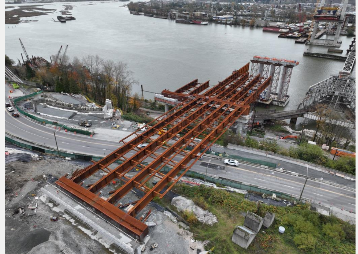
Photo 6: Ongoing girder installation for the North Approach
