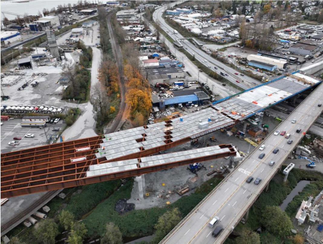
Photo 3: South Approach girder and deck installation
