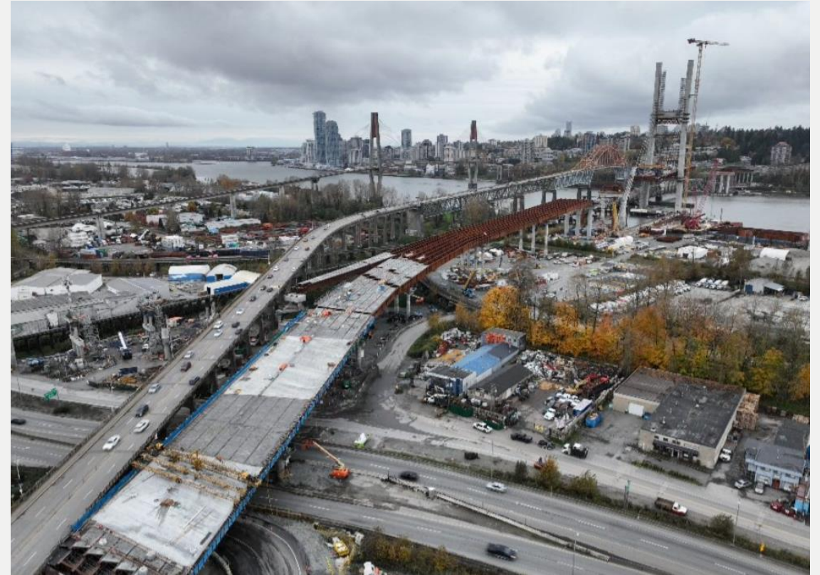
Photo 4: South Approach deck panel installation across Highway 17
