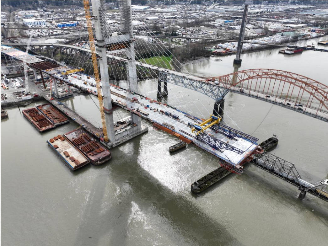
Photo 1: Main span construction south-west facing
