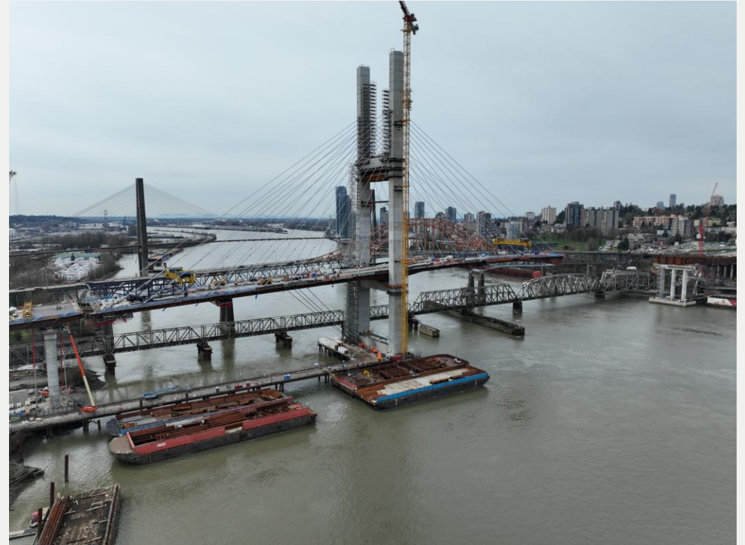
Photo 2: Halfway cable stays west facing
