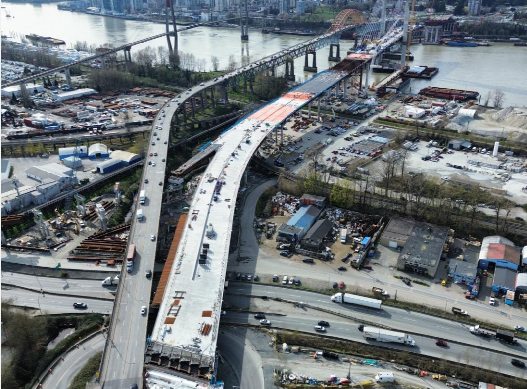
Photo 3: South Approach girder and deck panel installation
