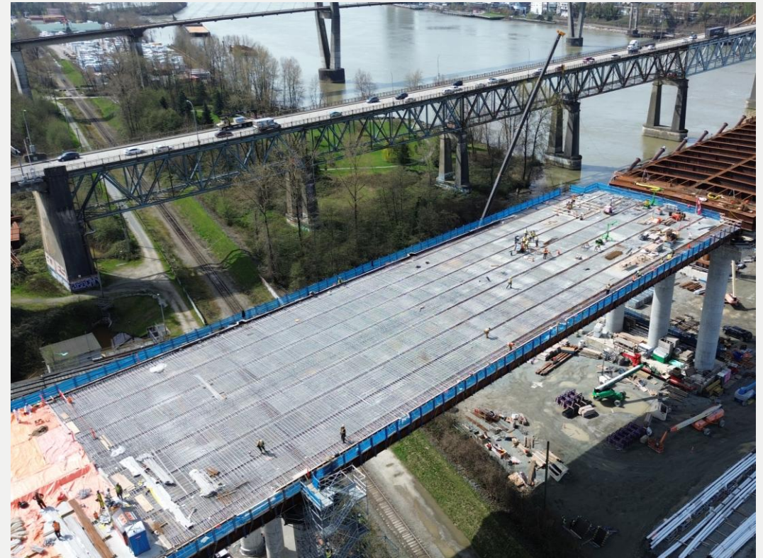
Photo 4: South Approach-Completion of deck panels
