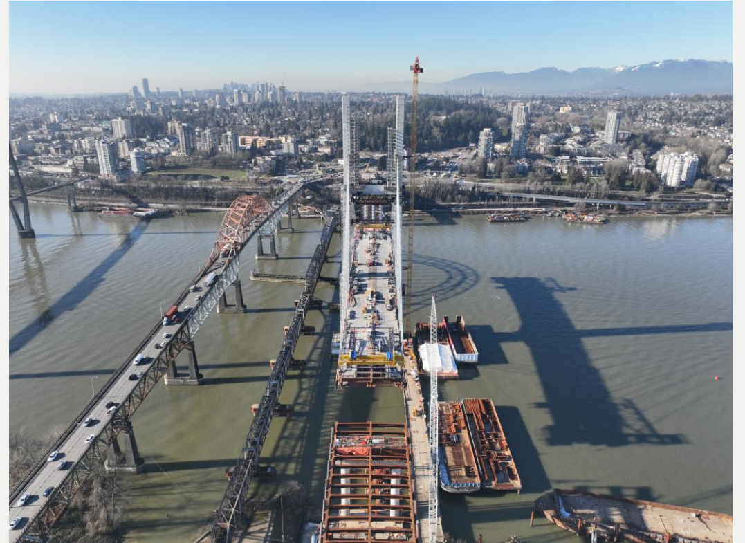
Photo 2: Pier S1, looking northeast
