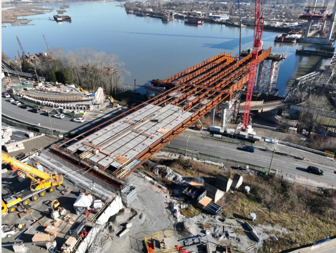
Photo 5: Ongoing girder installation at N1 Tower
