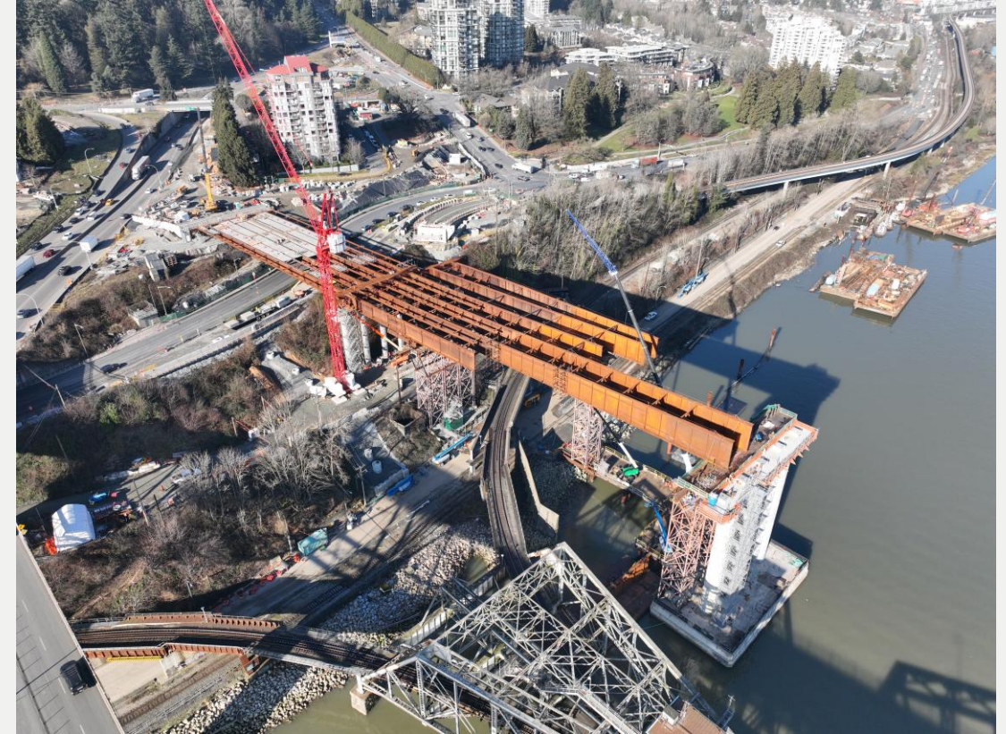
Photo 6: Ongoing girder installation for the North Approach
