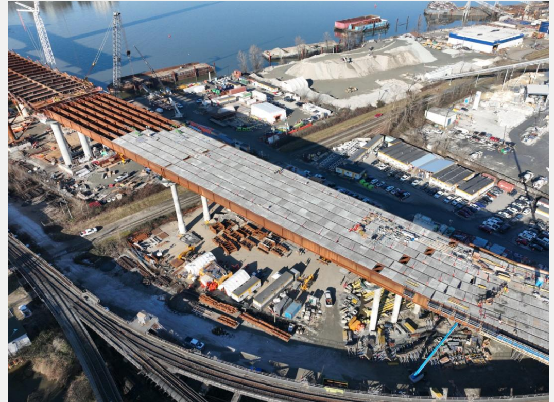
Photo 4: South Approach girder and deck installation
