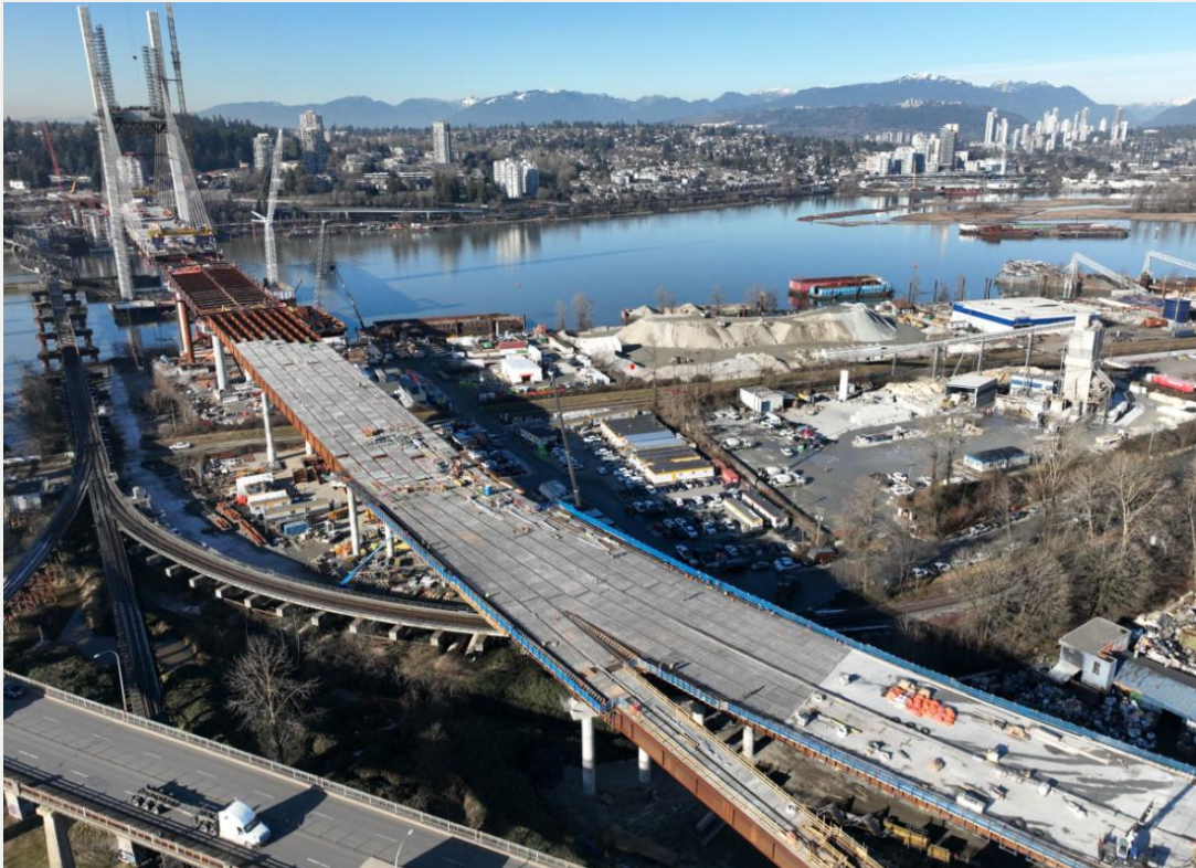
Photo 3: South Approach girder and deck installation
