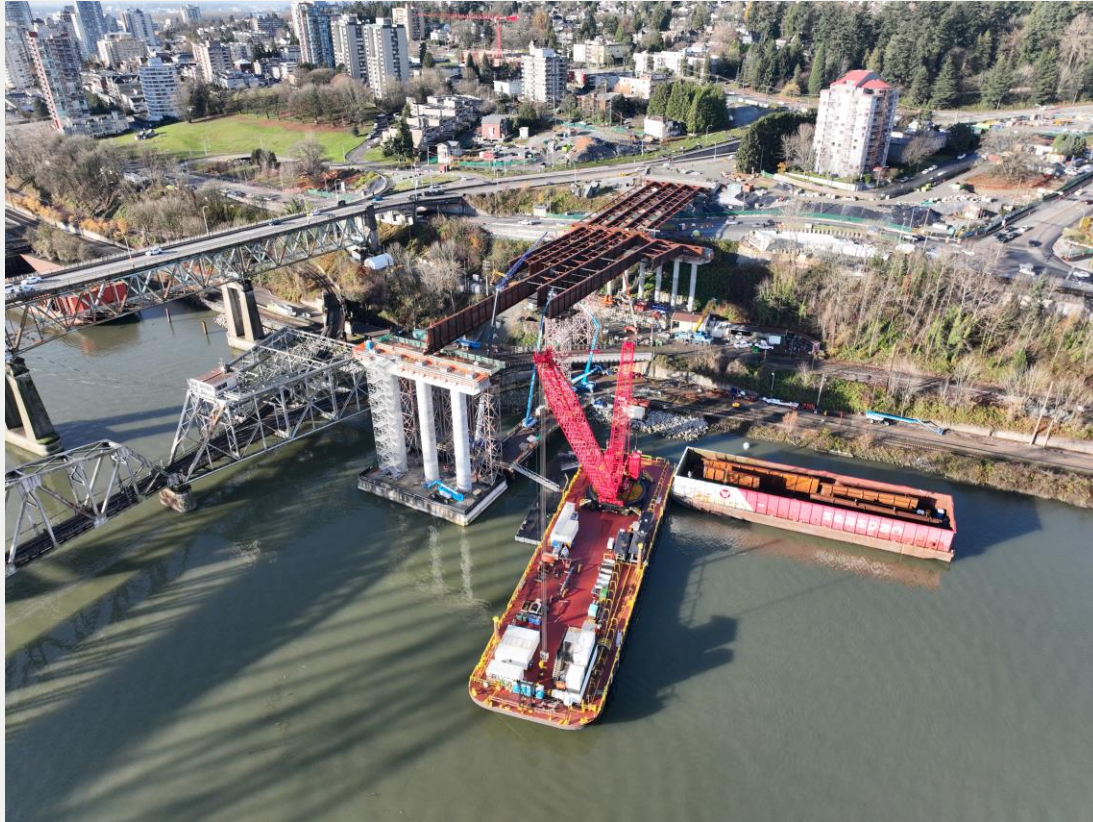
Photo 5: Ongoing girder installation at N1 Tower
