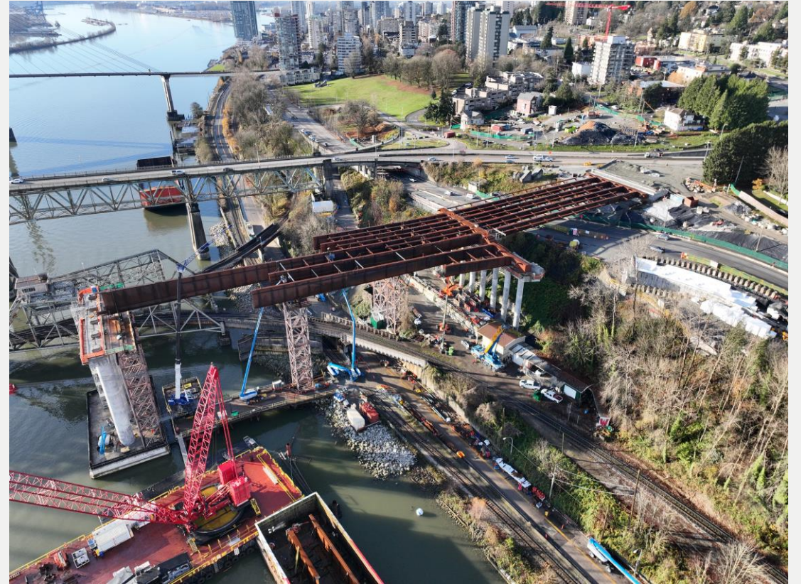
Photo 6: Ongoing girder installation for the North Approach
