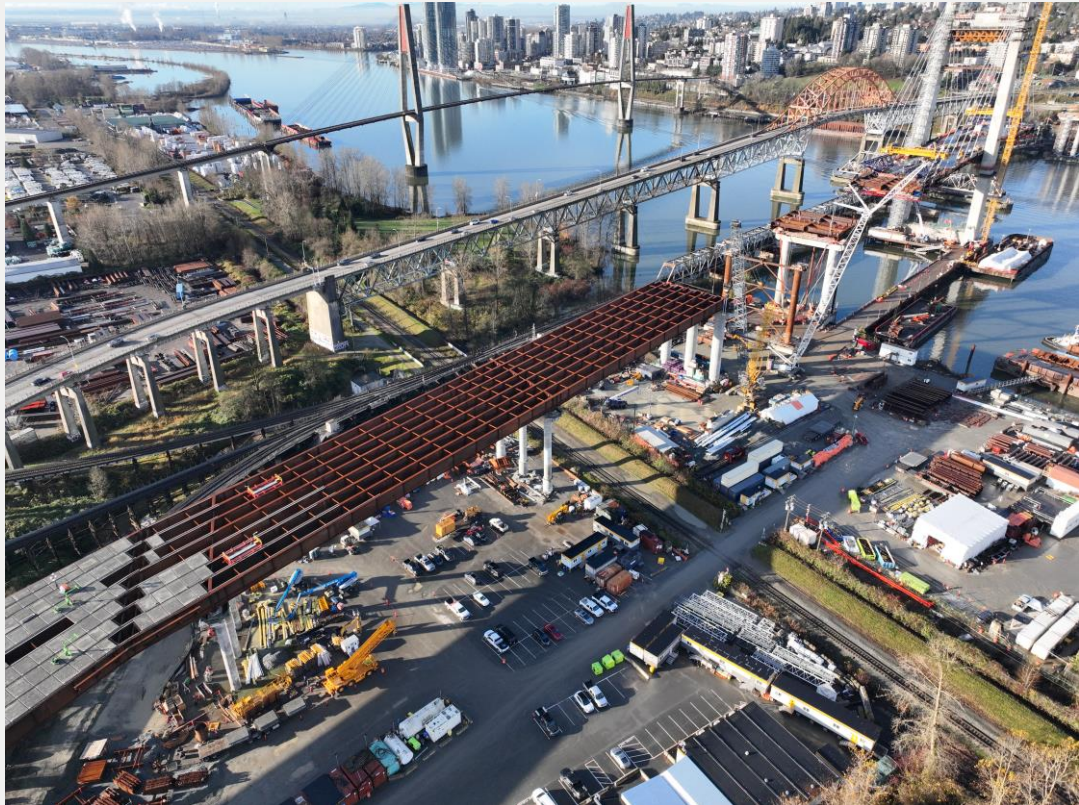
Photo 3: South Approach girder and deck installation
