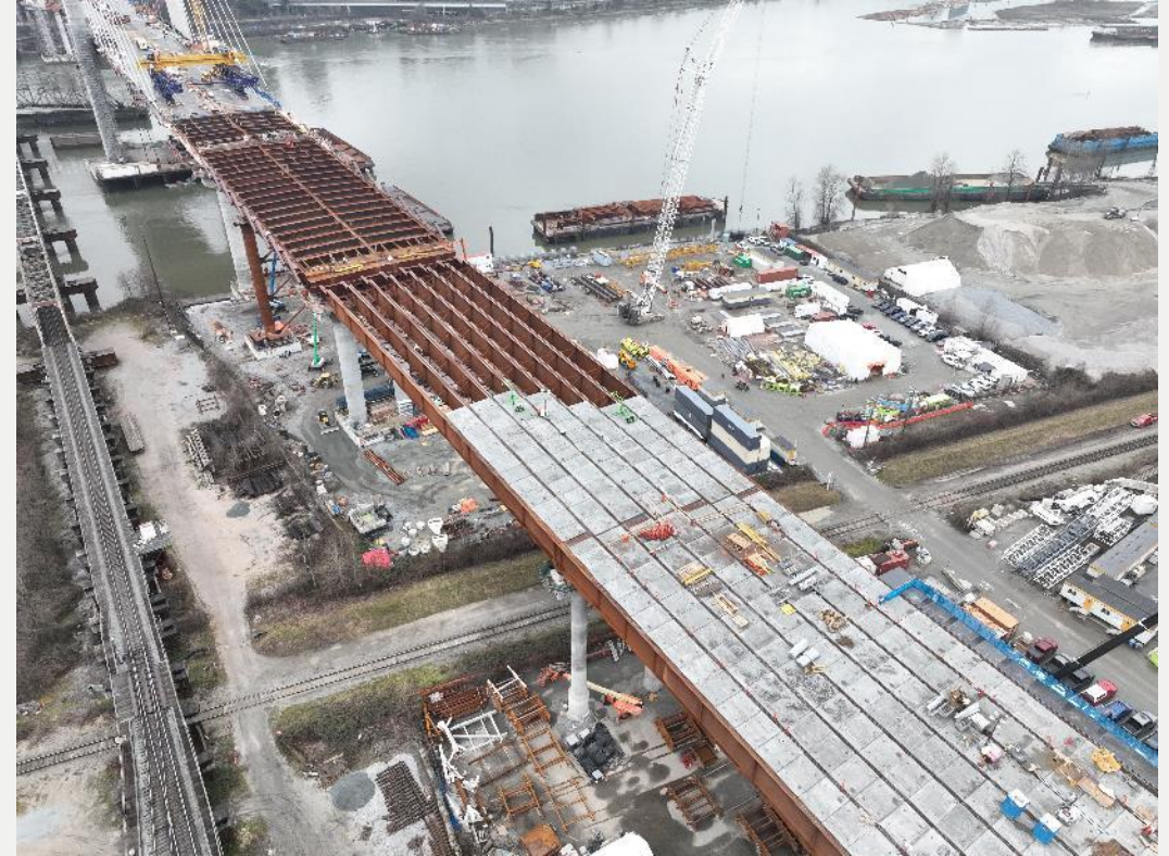
Photo 4: South Approach girder and deck installation
