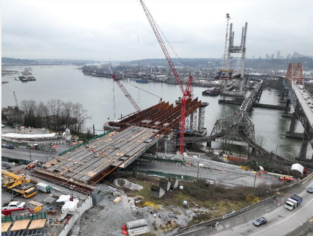
Photo 5: Ongoing girder installation at N1 Tower
