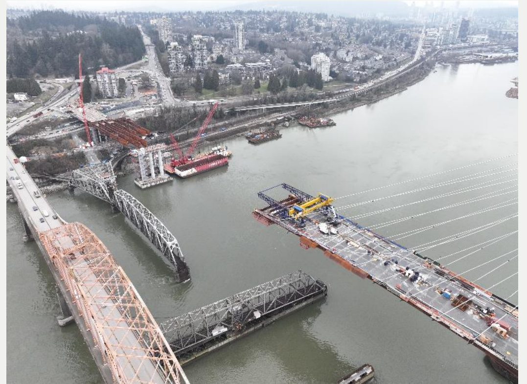
Photo 2: Pier S1, looking northeast
