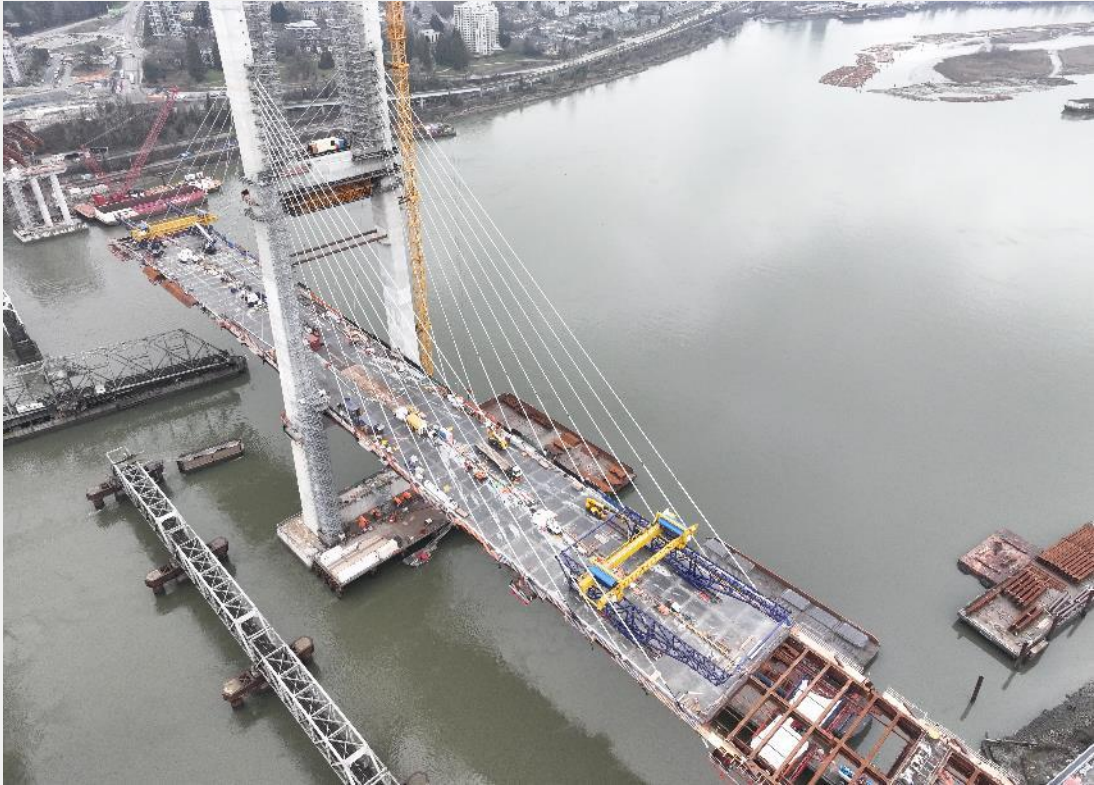
Photo 1: Pier S1, looking northwest
