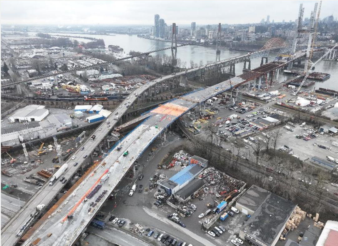
Photo 3: South Approach girder and deck installation
