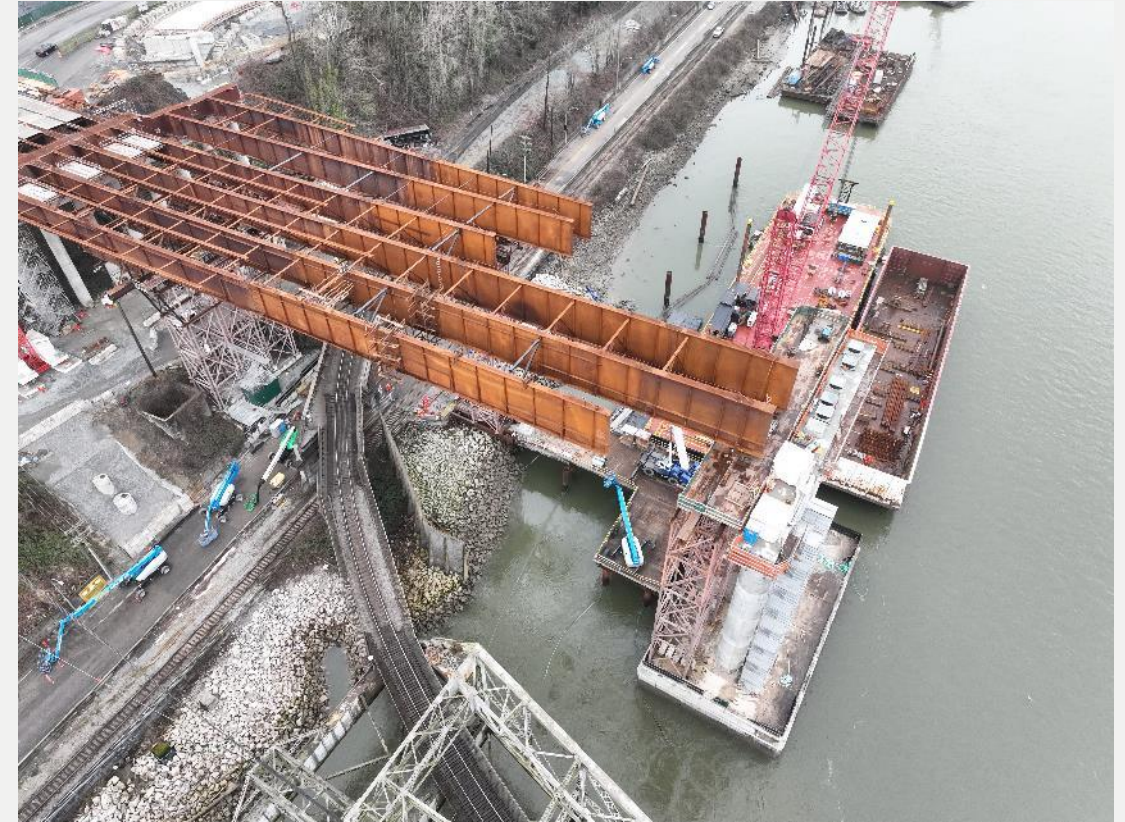
Photo 6: Ongoing girder installation for the North Approach
