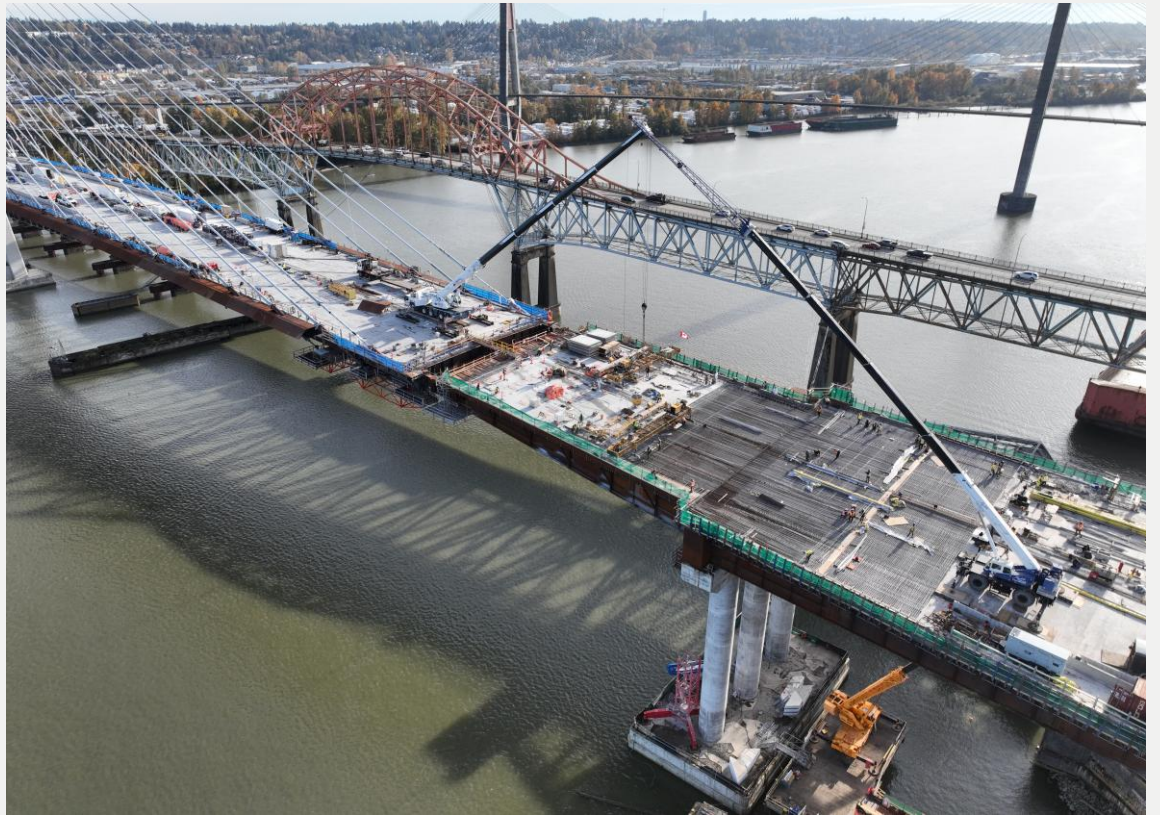
Photo 6: Main span almost connected to the North Approach
