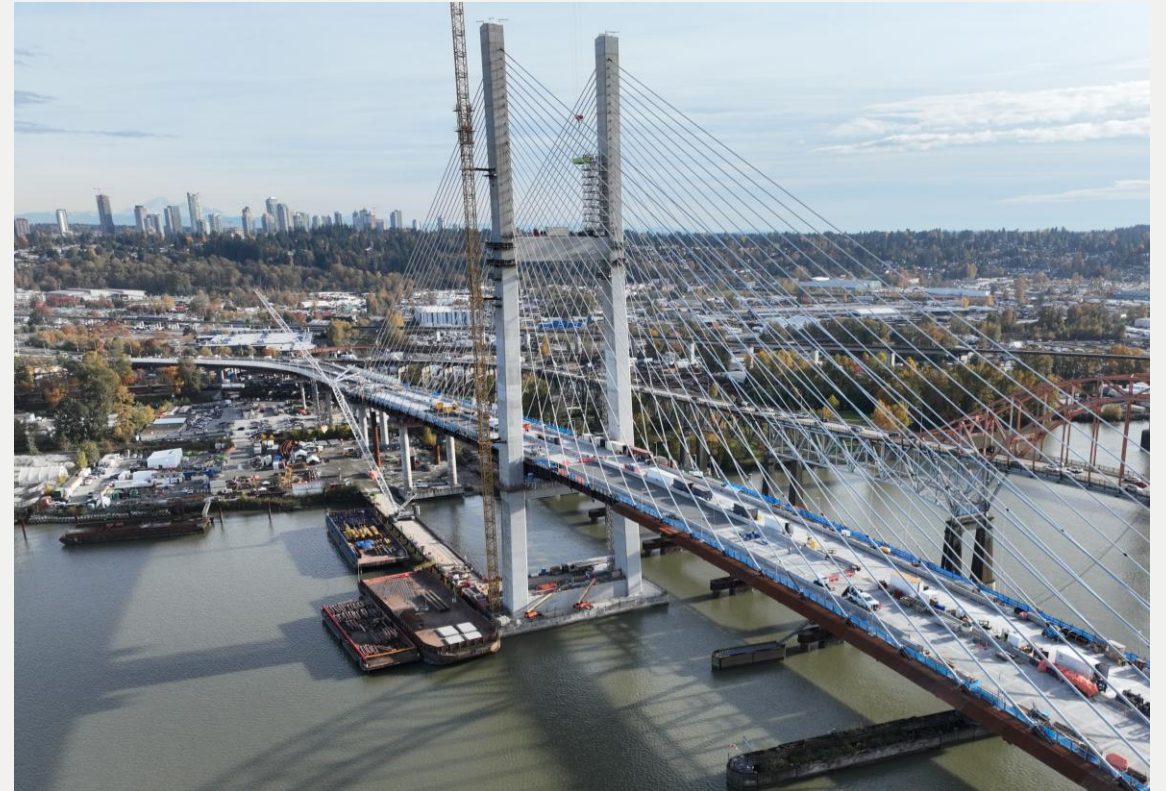
Photo 4: South Approach-end span and main span concrete overlay, finishings and paving ongoing
