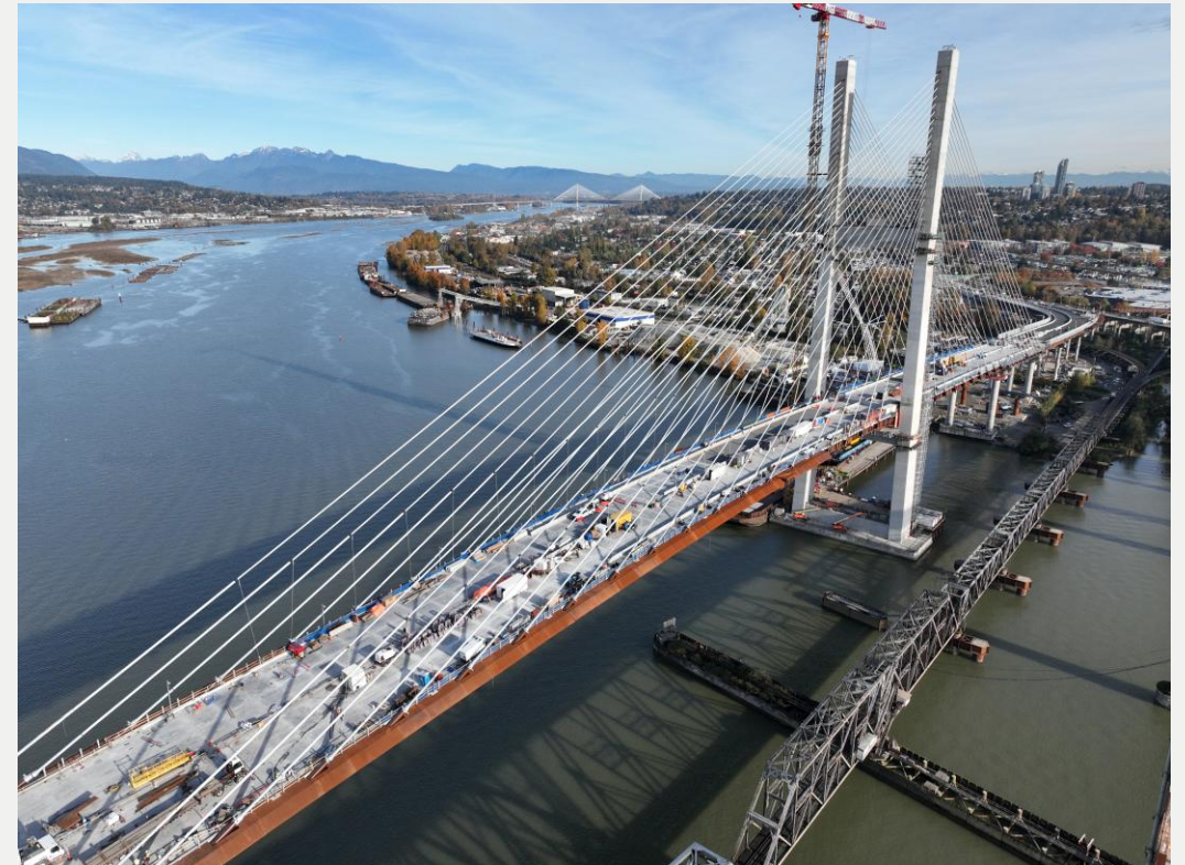
Photo 2: Bridge deck asphalt, cable stay, fence installation and other finishing works in progress
