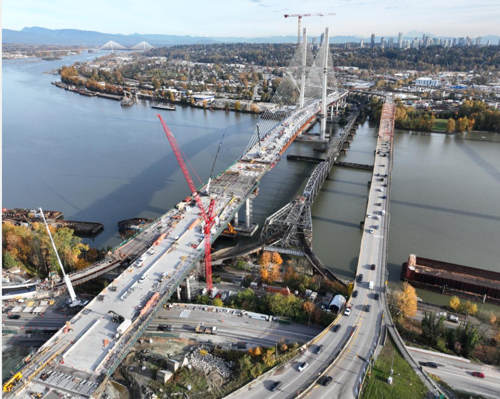
Photo 5: North Approach deck panels installation, deck pours, and concrete underlay works ongoing
