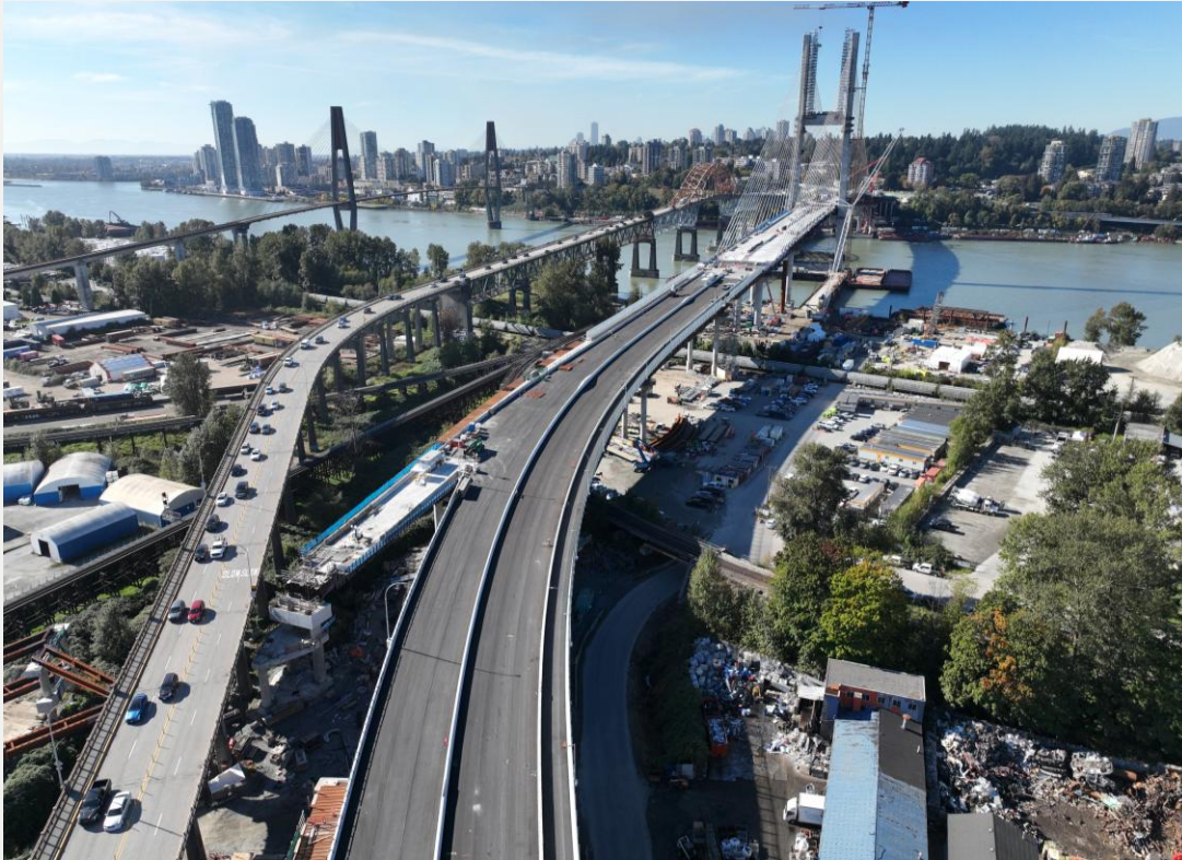
Photo 1: Bridge deck asphalt, cable stay, fence installation and other finishing works in progress
