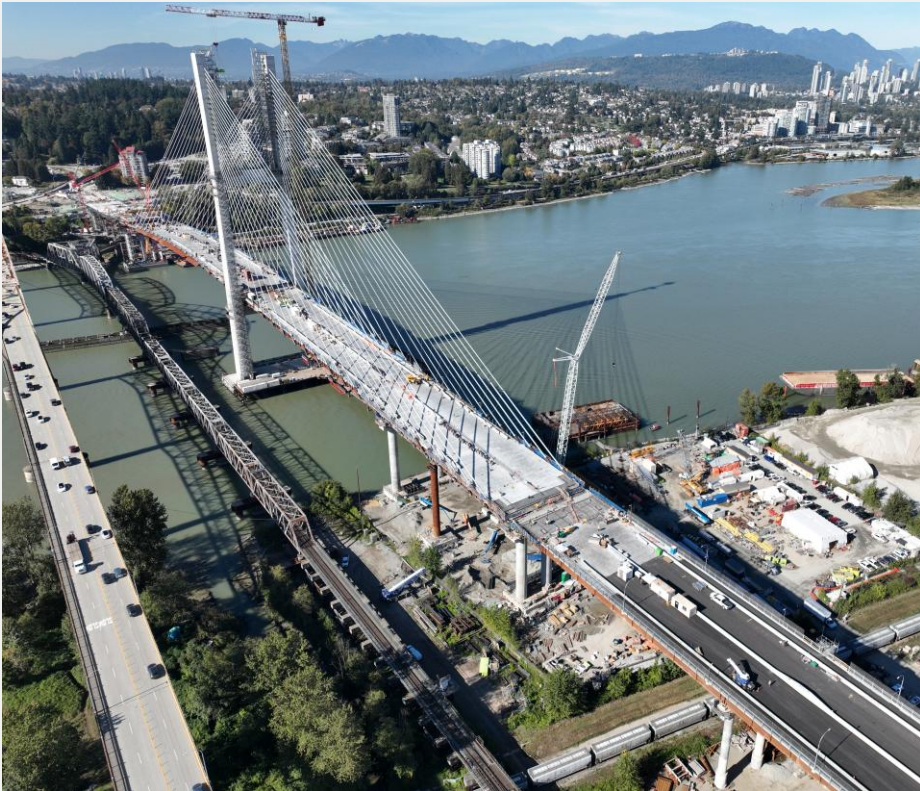
Photo 3: South Approach-end span- main span cable stay installation and finishing works ongoing
