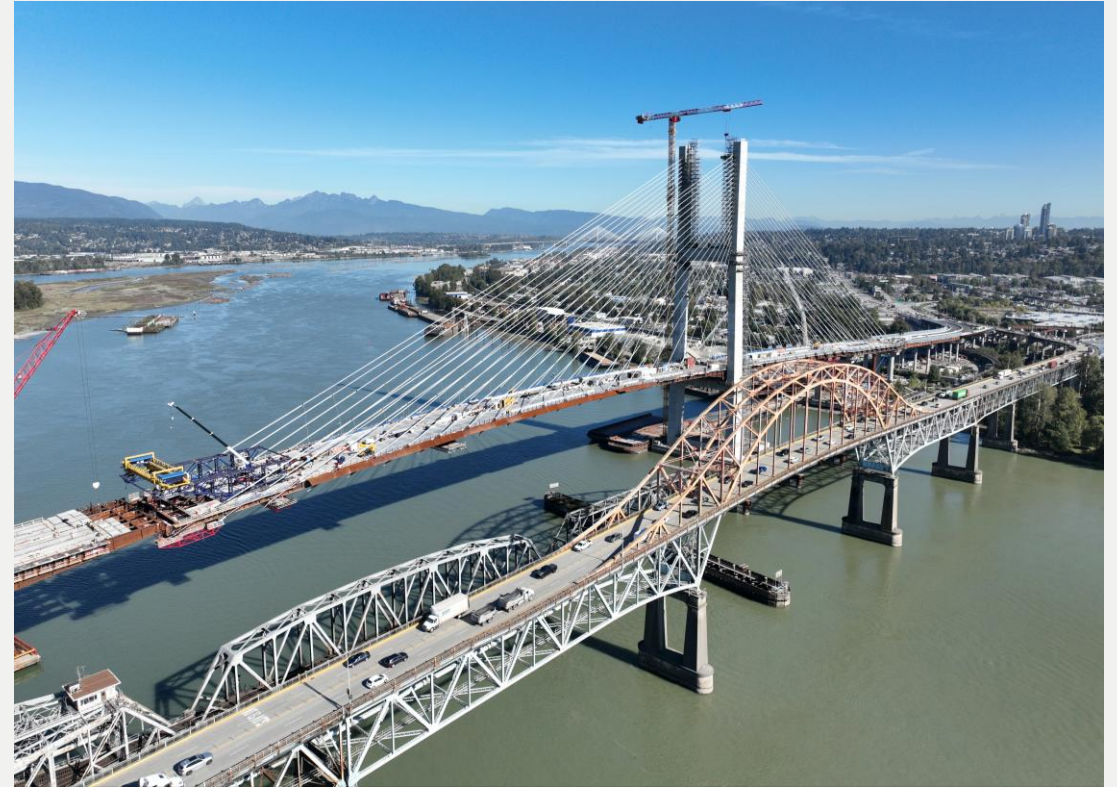
Photo 2: Main span and North Approach bridge connection works ongoing
