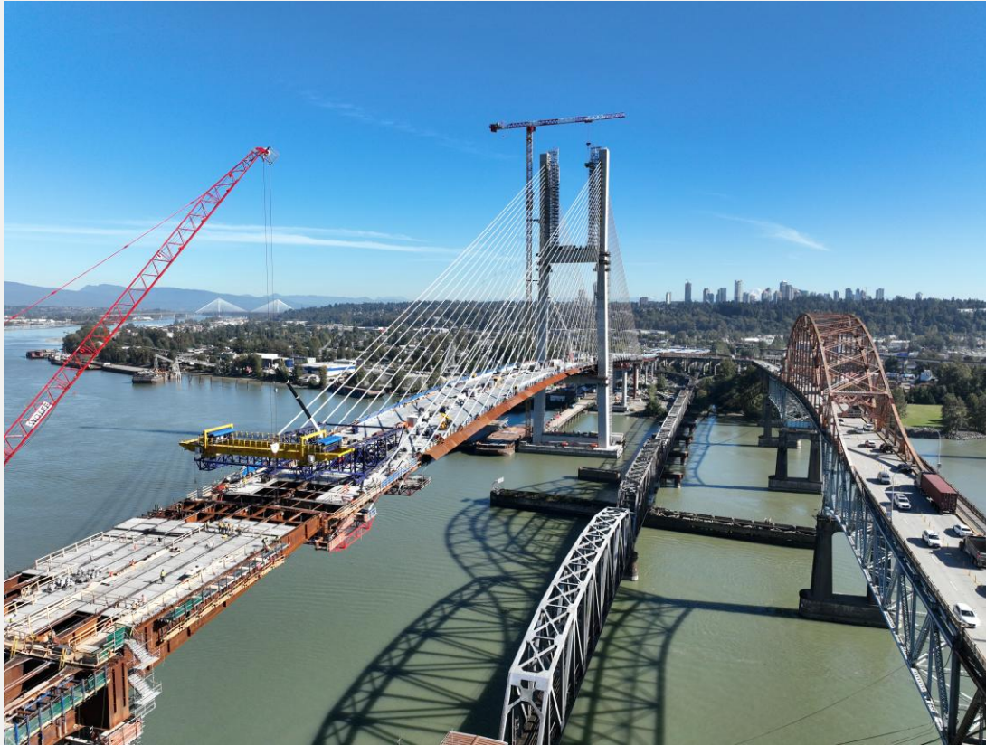
Photo 5: North Approach deck panels installation and deck pours ongoing
