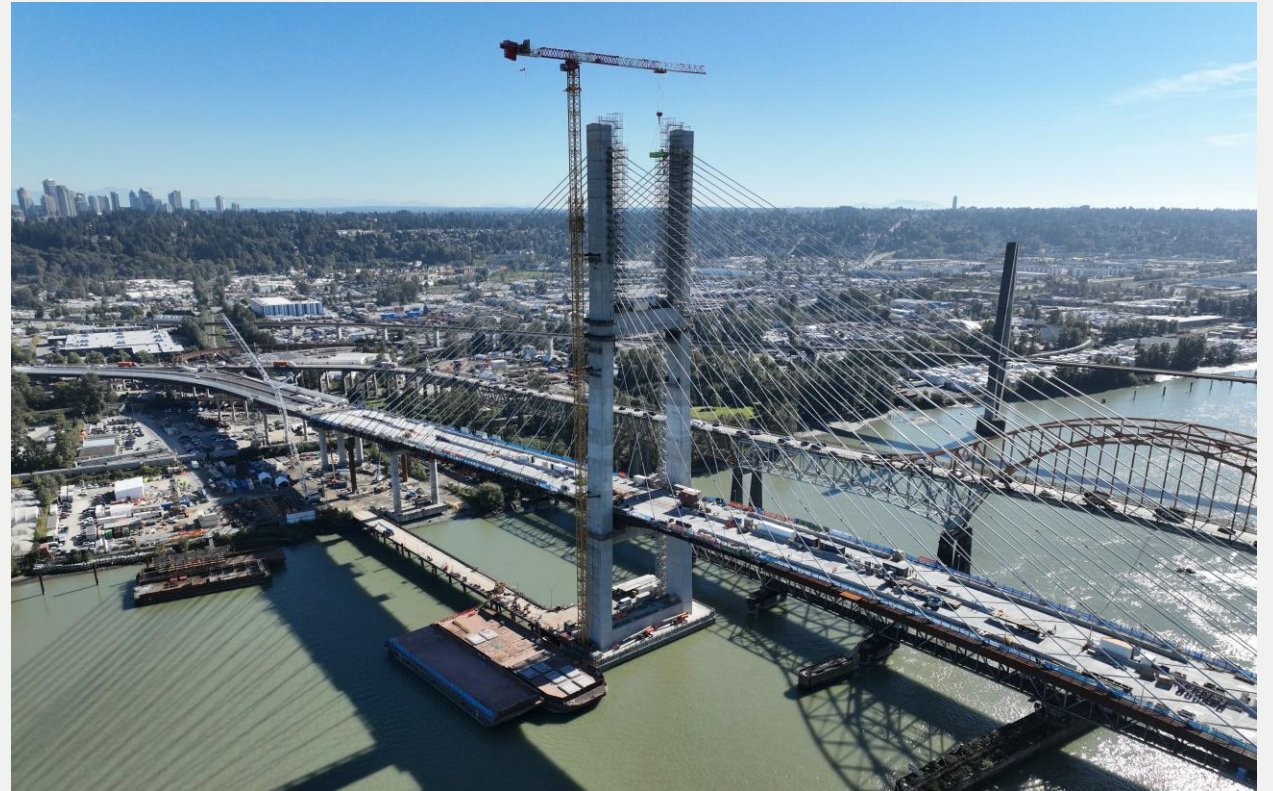
Photo 4: South Approach-end span and main span concrete overlay, finishings and paving ongoing
