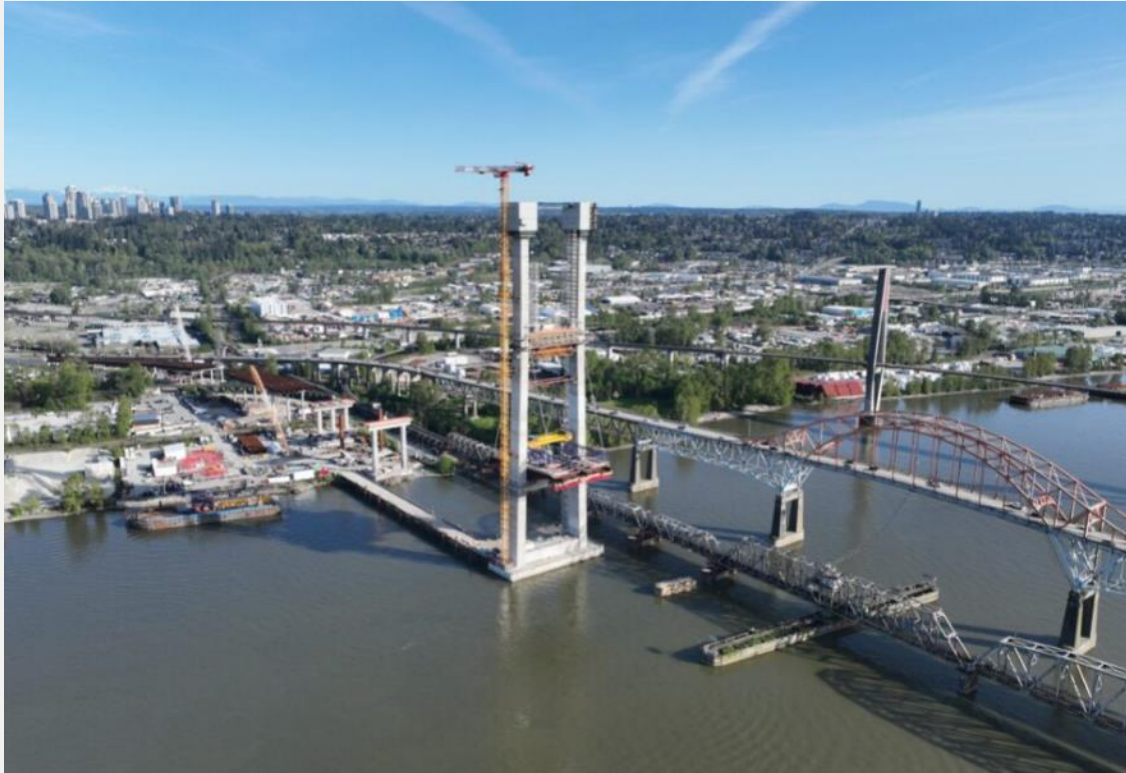
Photo 1: Pier S1, looking south
