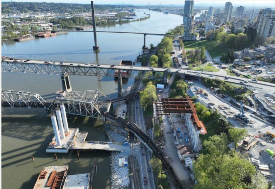
Photo 5: Pier N1 columns and girder installation at N2, looking west
