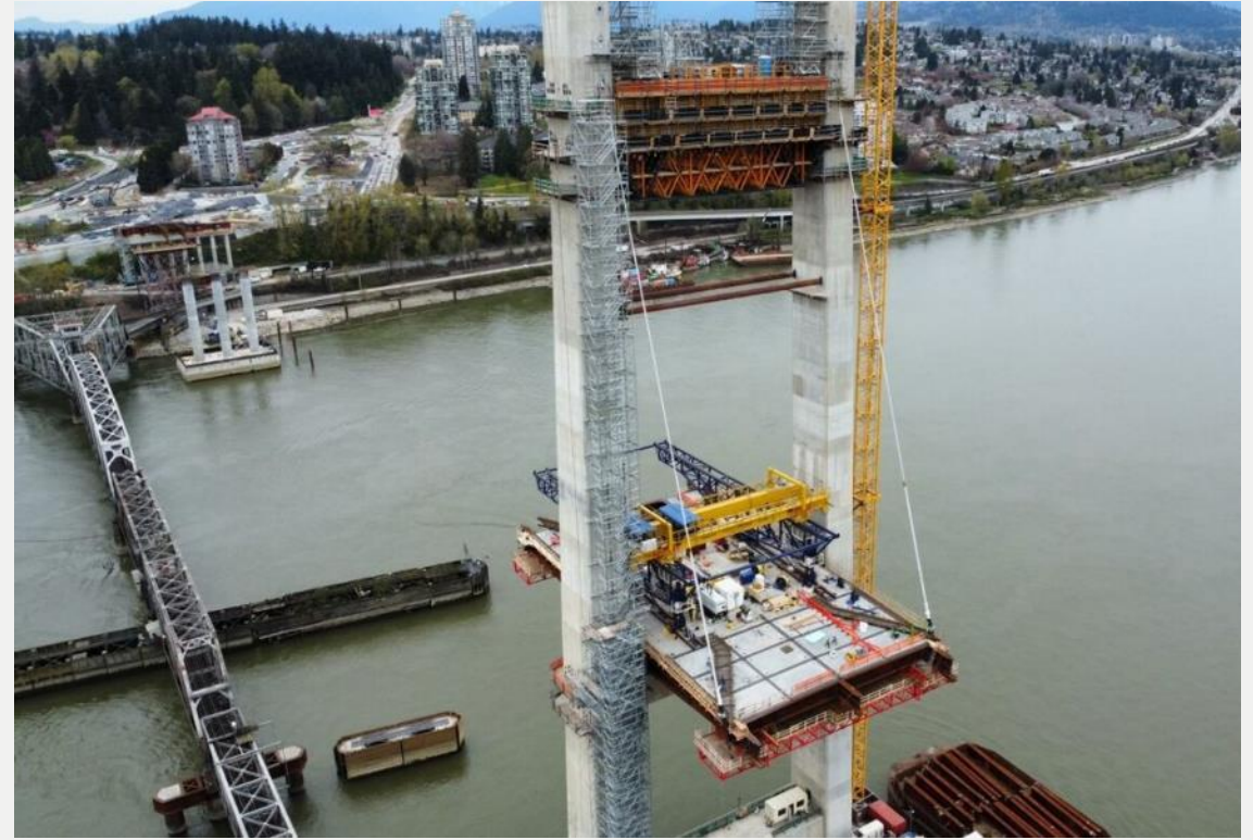
Photo 2: Pier S1, looking north
