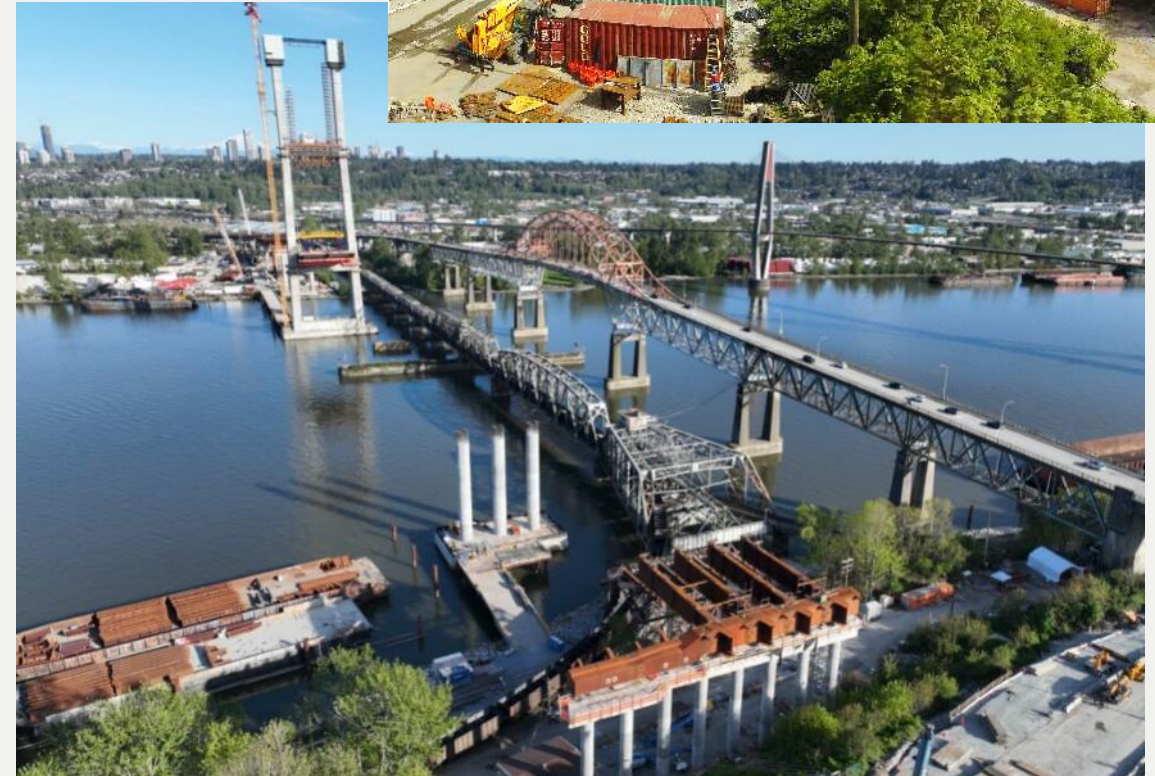
Photo 6: Pier N1 columns and girder installation at N2, looking south
