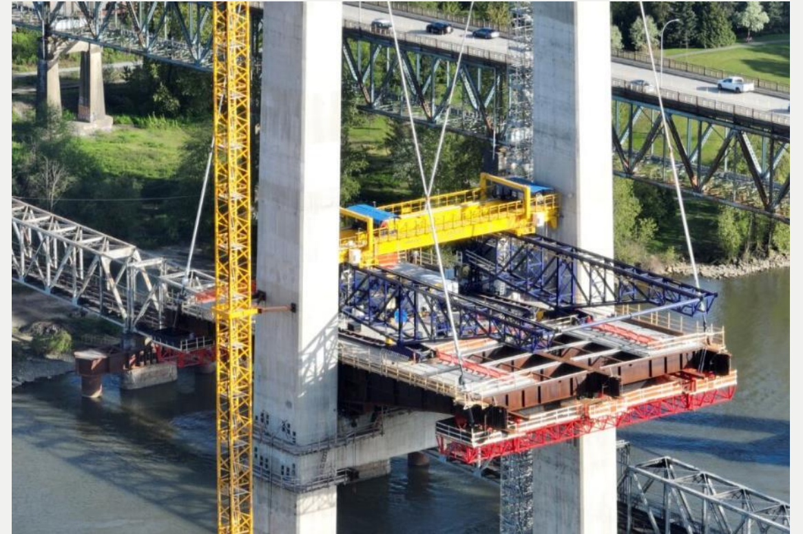
Photo 4: Bridge deck and cable stays, looking south
