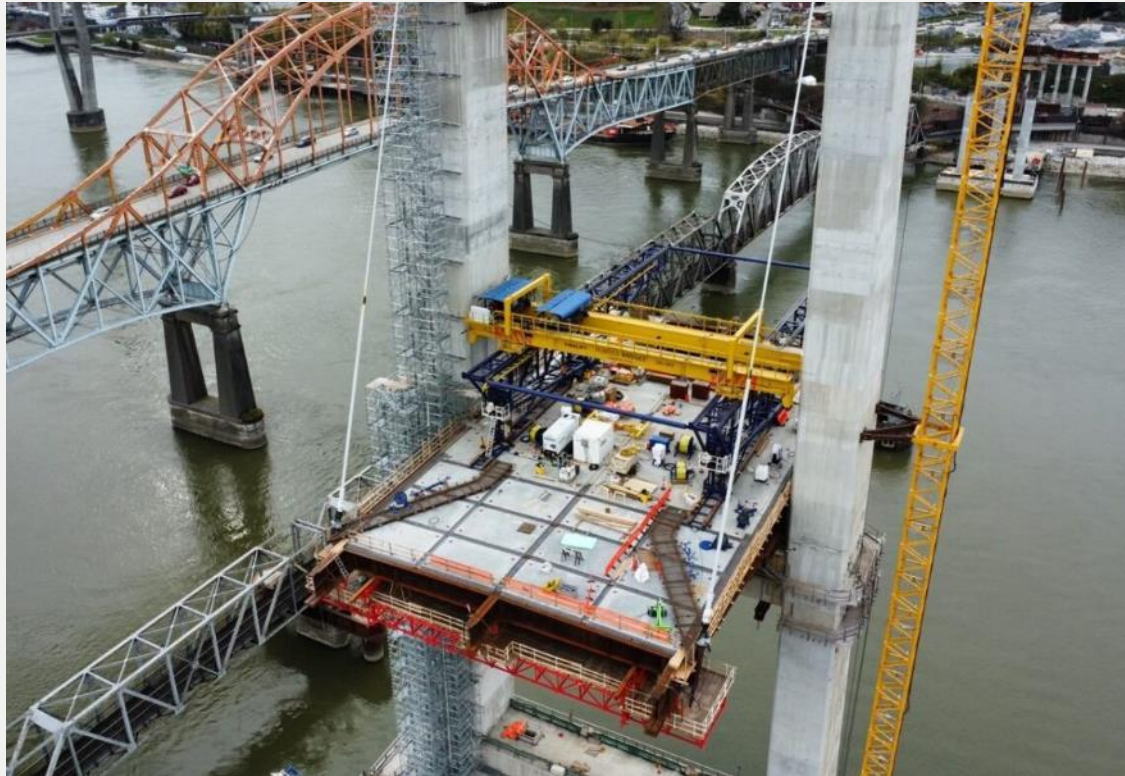
Photo 3: Bridge deck and cable stays, looking north
