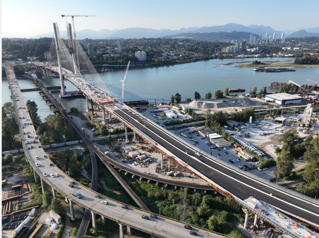
Photo 1: Bridge deck asphalt, cable stay and finishes in progress
