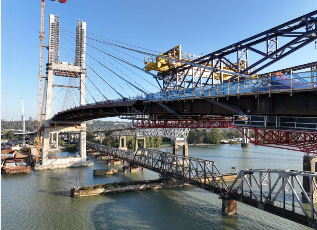
Photo 5: Main span bridge deck looking south with Rolling Skyline platform
