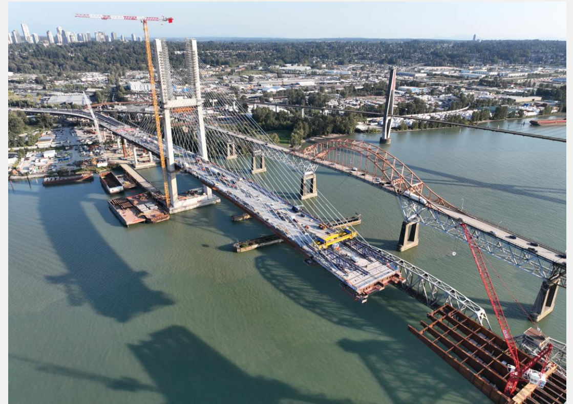
Photo 2: Concrete overlay on bridge deck and connection to North Approach ongoing
