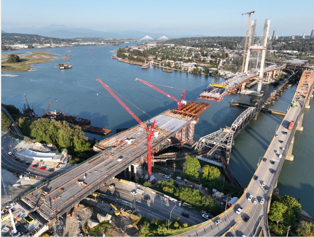
Photo 7: North Approach deck panels installation and deck pours ongoing
