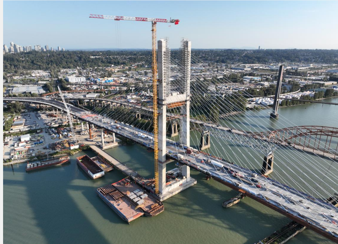
Photo 4: South Approach-end span and main span concrete overlay, finishings and paving ongoing
