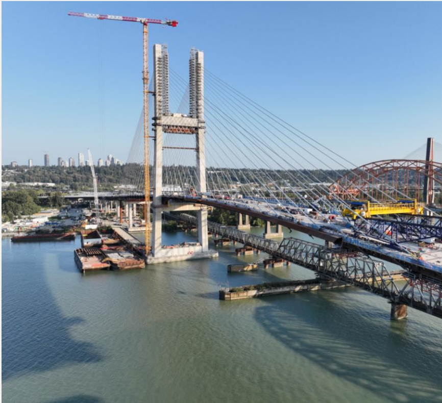
Photo 3: South Approach-end span- main span cable stay installation and finishing works ongoing
