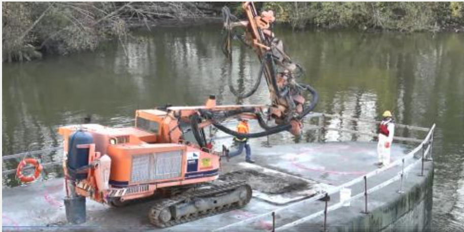
Typical arrangement of drilling holes for placing explosives
