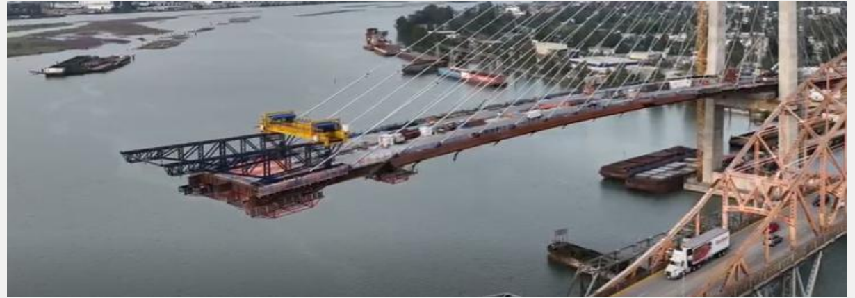
Photo 6 above: Underslung platform located at the northern tip of the main span. Photo 7 below: Illustration of the rolling track used by the skyline gantries
