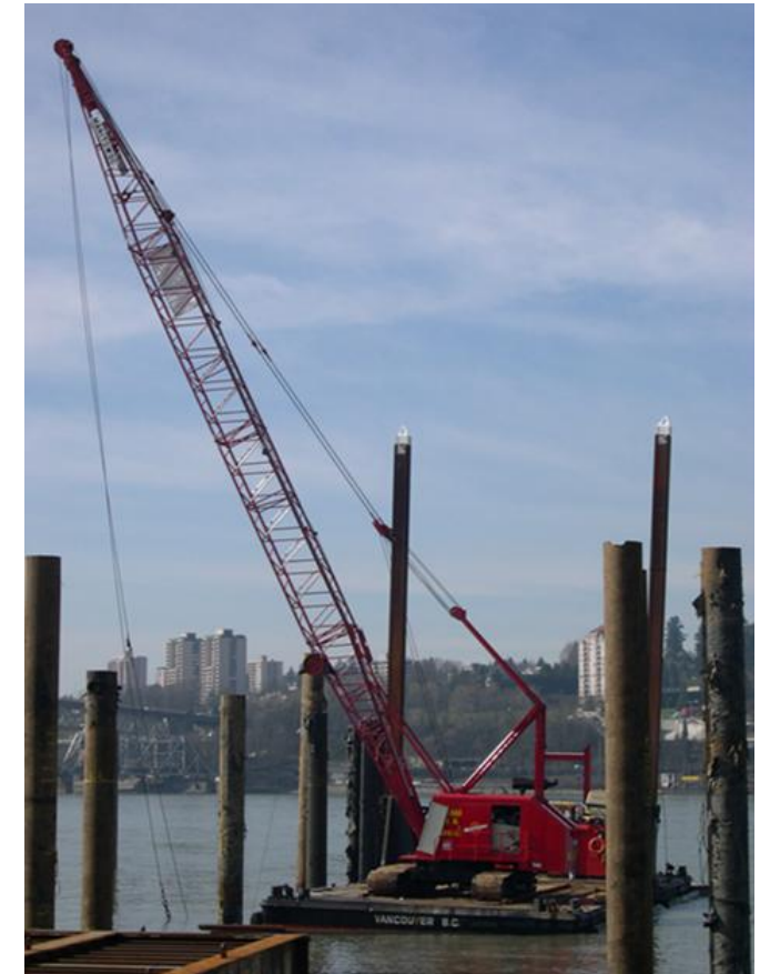
Derrick Barge FRPD GE#6 (LOA 28.3m beam 12.5m x draught 2.1m)
