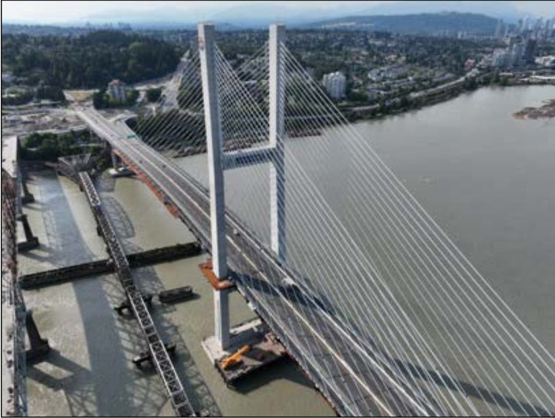
Photo 1: Bridge finishing works ongoing including installation of safety fence and artwork installations
