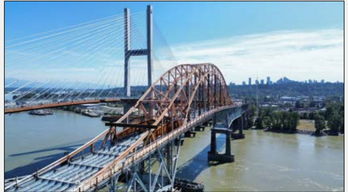
Photo 4: Vertical props and columns to support Span 4 (arch) lowering installed along Span 4
