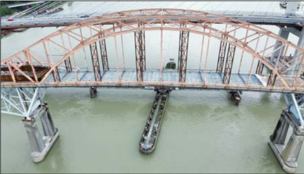
Photo 5: Span 4 bridge deck removal complete
