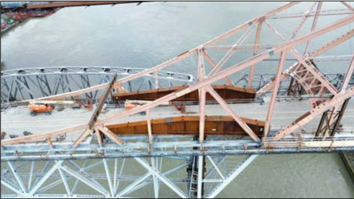
Photo 3: Installation of the Pier P3 jacking box beams and frame
