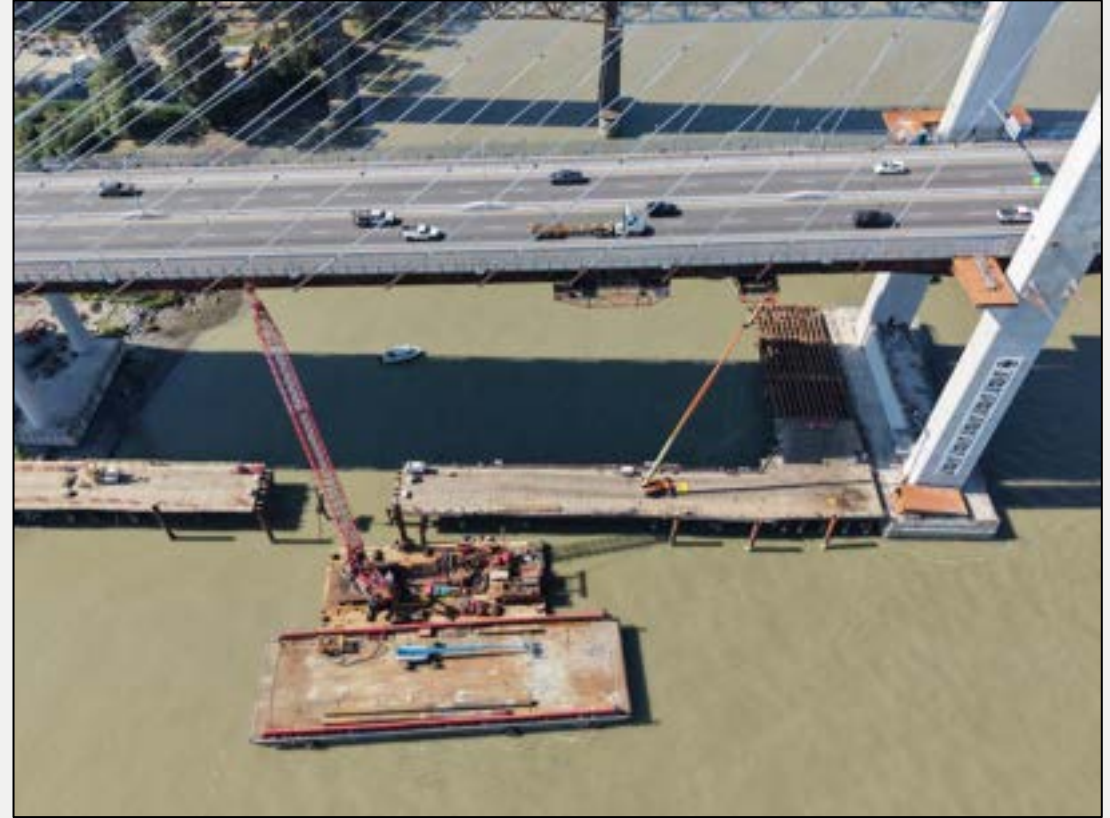
Photo 2: Pier S1 Temporary Work Platform (TWP) removal in process
