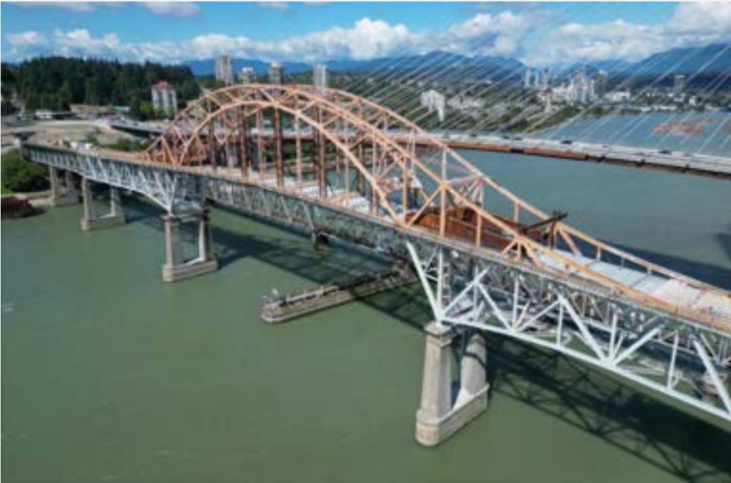
Photo 5: Span 4 and 5 bridge deck removal complete
