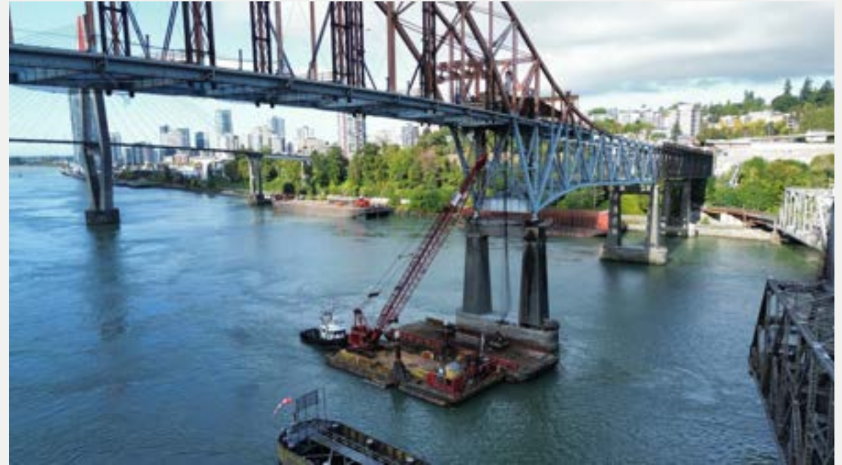
Photo 6: Span 4 lowering beam installation
